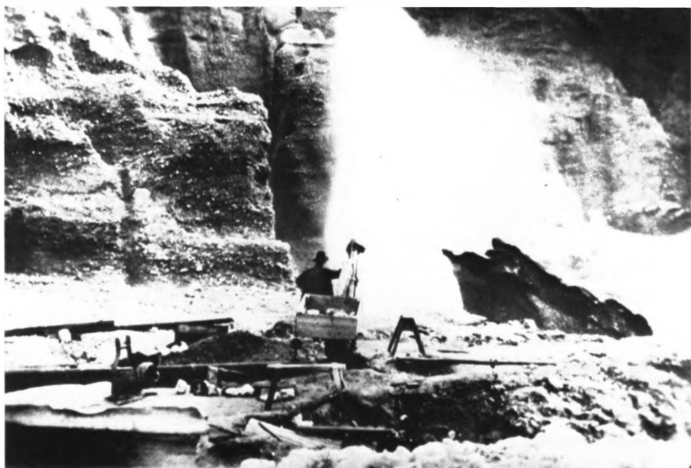
40 Placer mining in the Klondike. Gold-bearing gravels were washed out using a powerful jet of water. A similar technique, sometimes called hushing, was used by the Romans in Spain
